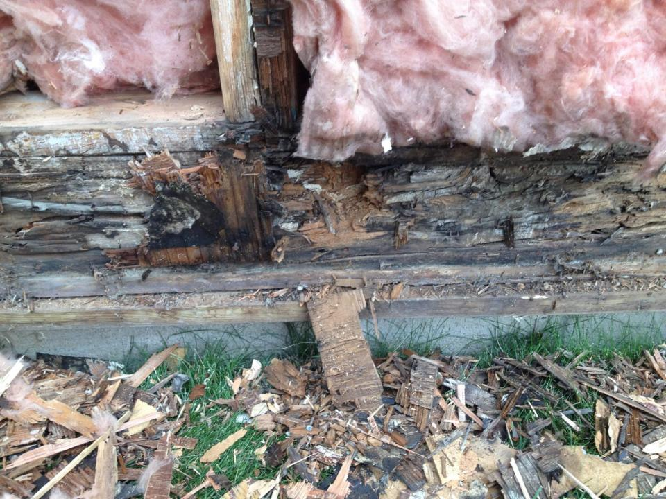
Carpenter Ants were found to have damaged many units, pest control was called at all locations with active issues. Site grading caused water and snow to move towards the buildings and was a large factor in causing floor structure rot.
